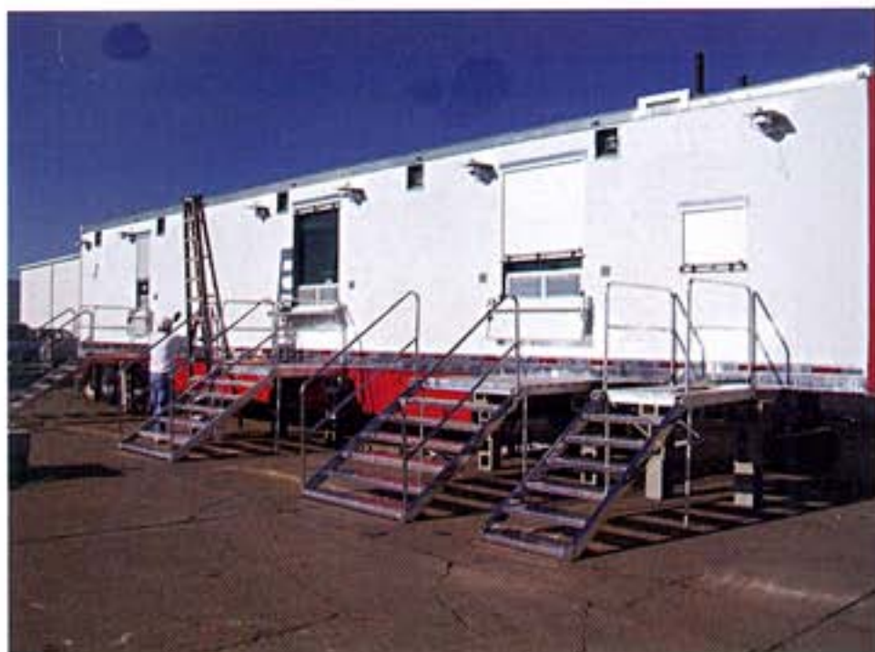
A view of the H-E-B disaster-relief trailer during construction ...
